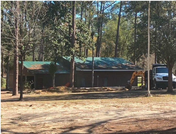
Figure 1: Demolished Old Amphitheater
