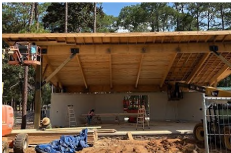
Figure 1: The Fulwood Park stage construction progress as of 8.14.2025
